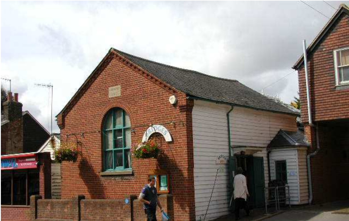
2. Historic ~Listed Chapel - now a community centre
