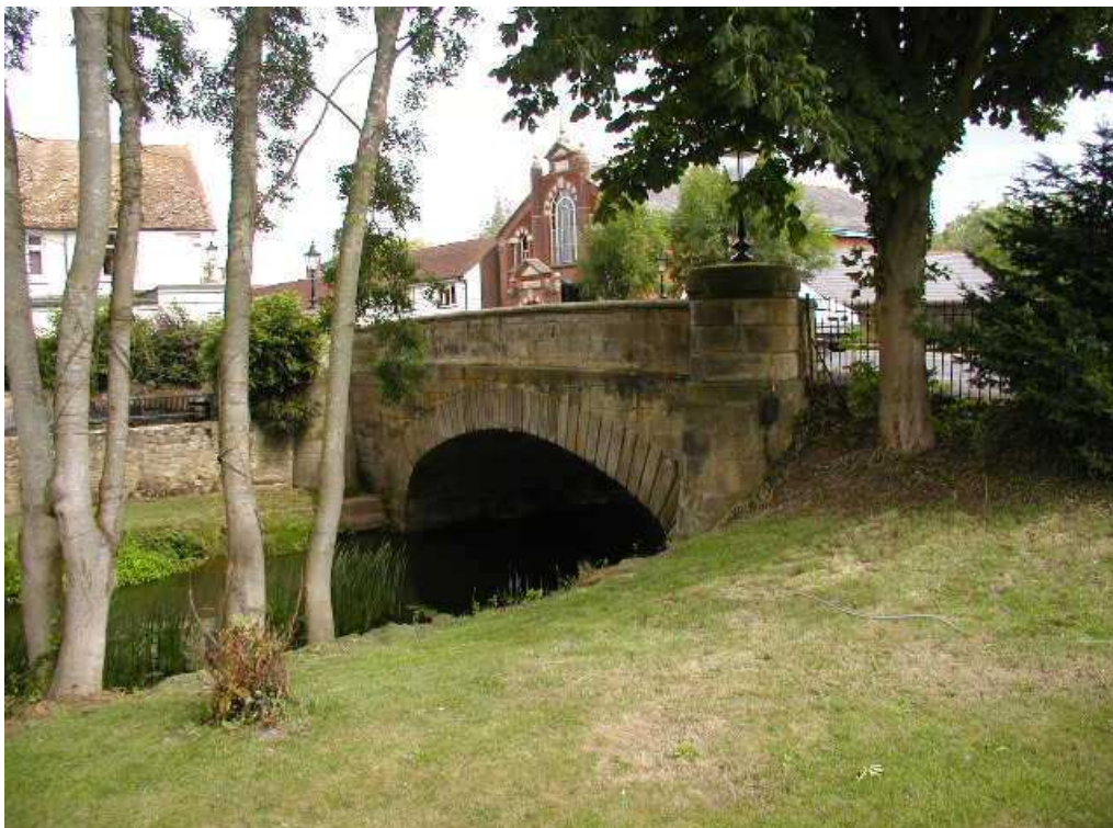
86. The Great Stone Bridge is a key historic feature within the Conservation Area.
