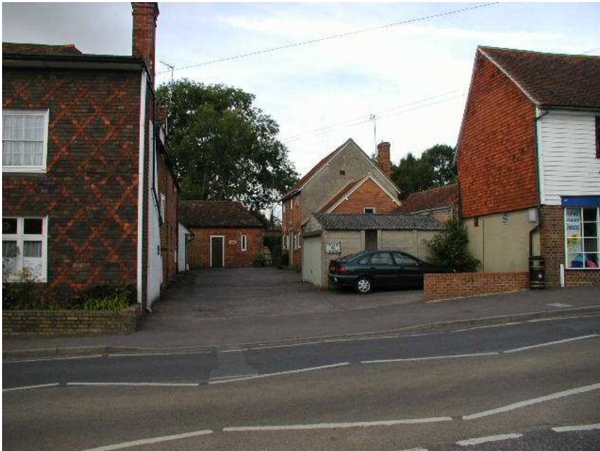
36.yard to no.2 High Street
