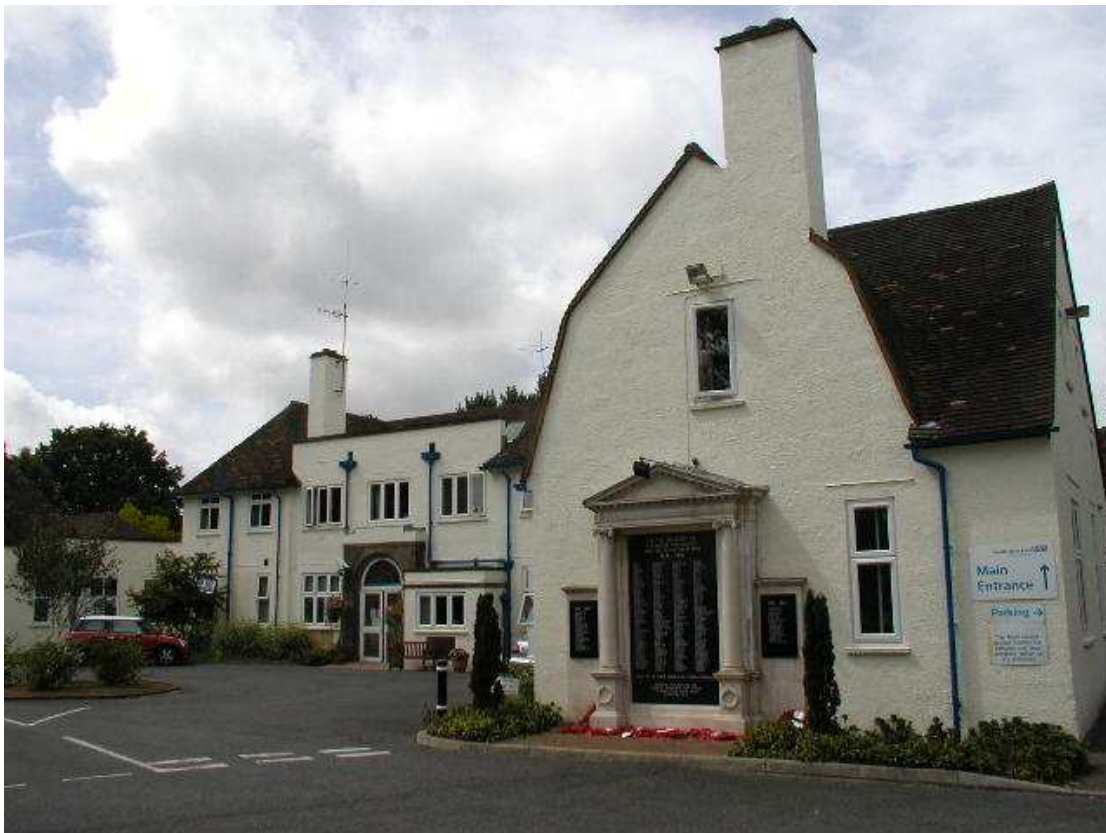
74. This 1930s cottage hospital is suitable in size and scale and of noted historic interest, by Mr H Read of Read and Macdonald, 1928-1931
