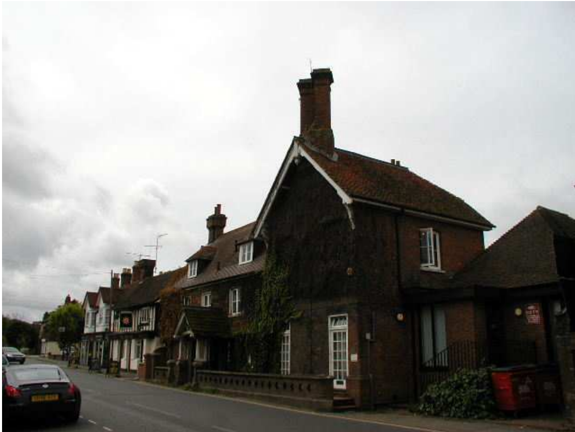
29. Edenbridge House - later additions hide an older timber framed structure
