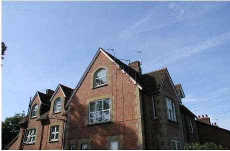
82. Unsightly clutter of aerials facing the highway
