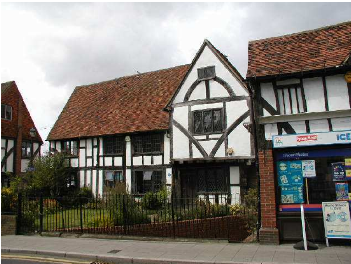
28. Typical Timber Framing to nos. 92 -94 High Street
